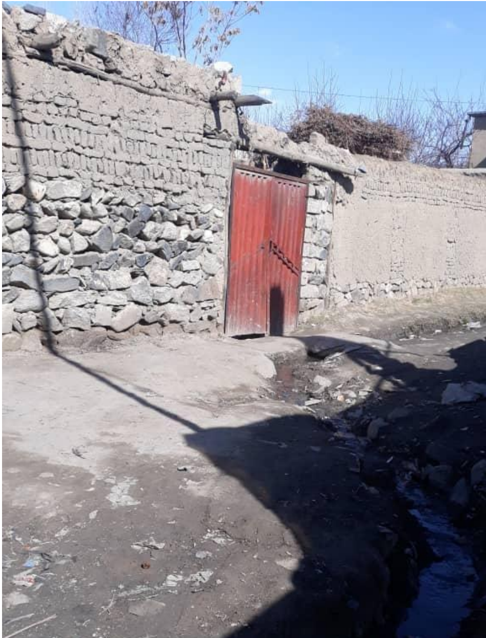
house of Masoom Allah Varduji
